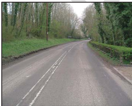
Worn road markings (WEAR)
