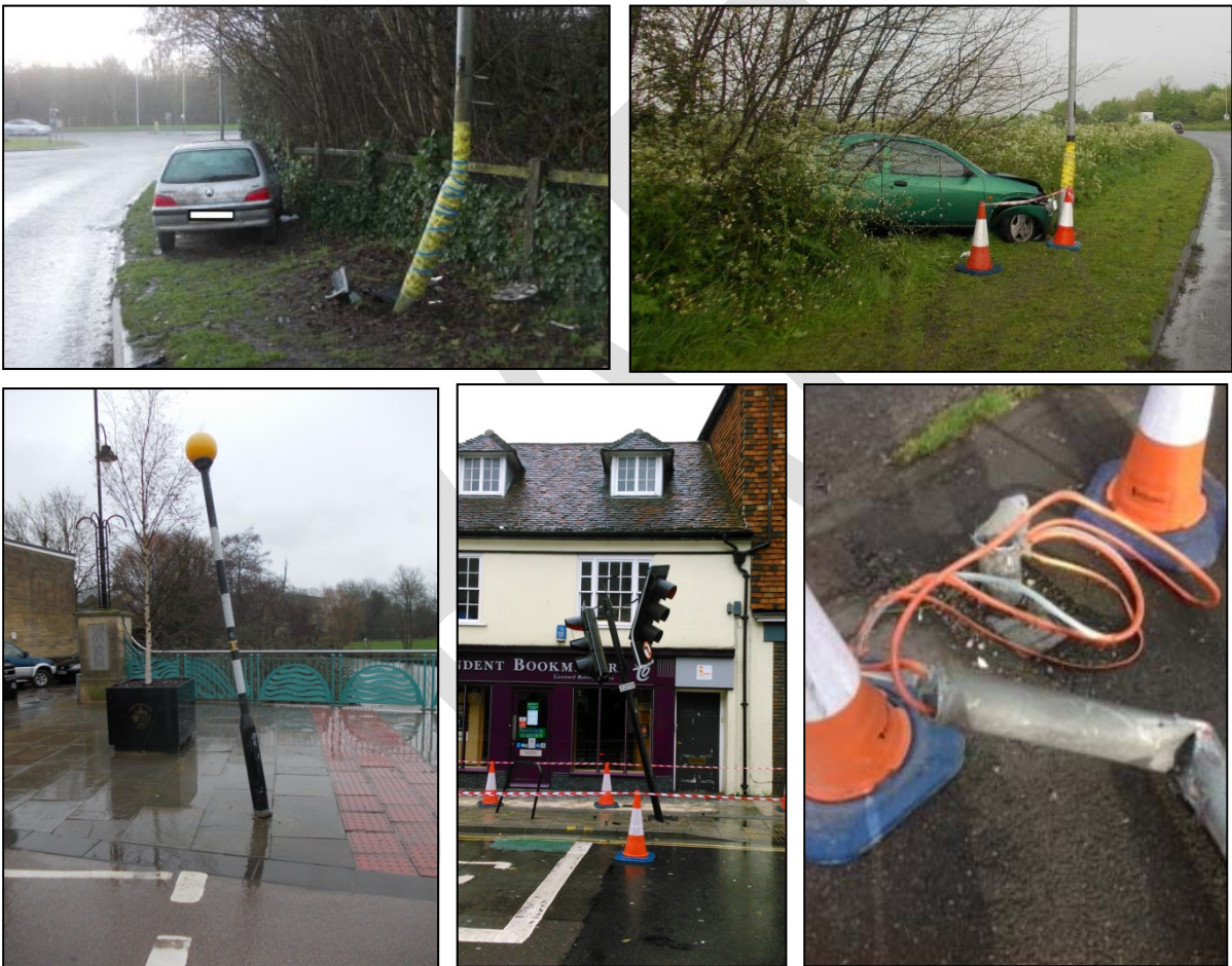
Damaged electrical installations and equipment (LIGH)
